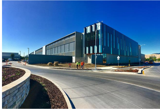
Figure 5: Equinix SV5 San Jose Data Center
