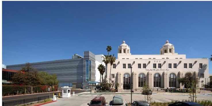
Figure 6: LA3 CoreSite Data Center in Los Angeles
