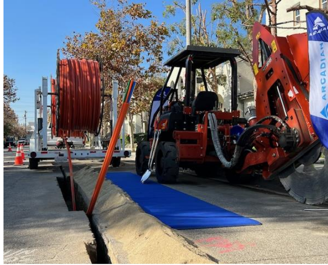
Figure 6: Microtrenching to install conduit
