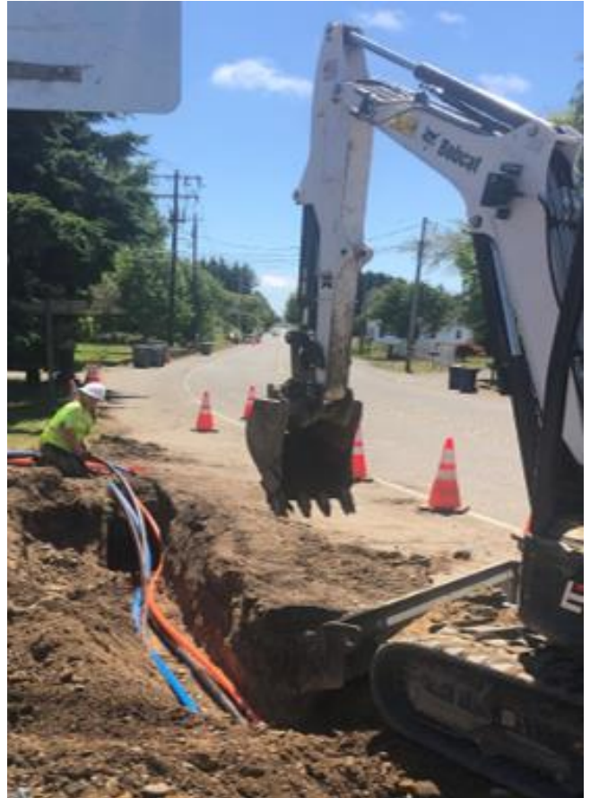
Figure 2: Construction trench with conduit
